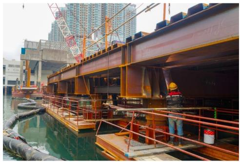
5. Given the limited workspace for construction along the Tuen Mun River bank, the project team is building a temporary river-crossing access for the delivery of construction materials.
